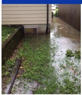
Stormwater runoff emanating from eight (8) residential lots located north and east of this location flows to the rear of the property where it is impeded by physical barriers and the yard grade. The runoff is frequently excessive and has entered a rear basement window of the home on several occasions. There is minor yard erosion evident in some areas of the rear and side yard.
