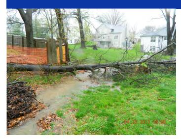
Stormwater runoff from a large drainage area roughly bounded by Eldon Avenue on the west, Midland Avenue on the south and Edgeworth Avenue on the east is conveyed across the property at 2860 Hathaway Avenue. The volume of runoff is sizeable and has eroded the lawn along a rear fence on the property and the perimeter of an area inlet that receives the flow at 2808 Hathaway Avenue.
